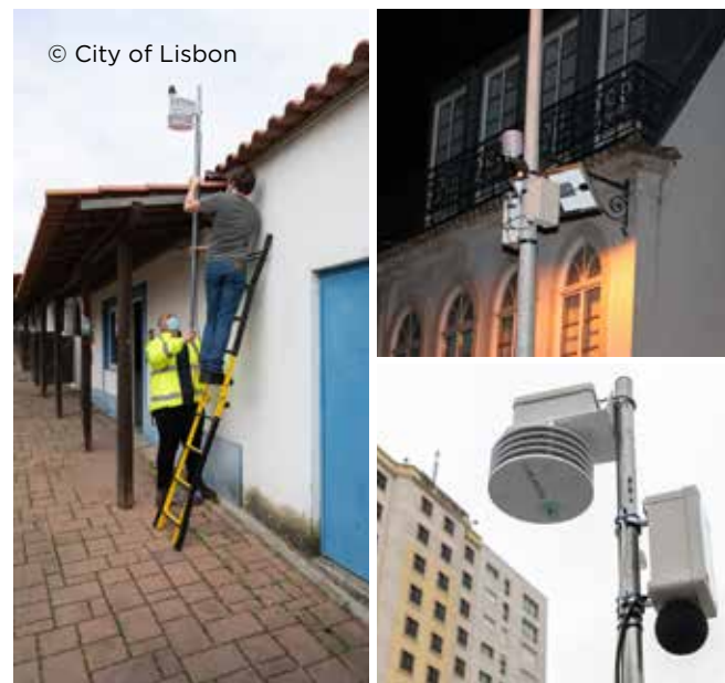
Figure 12: Sensor locations on light poles in Lisbon.
