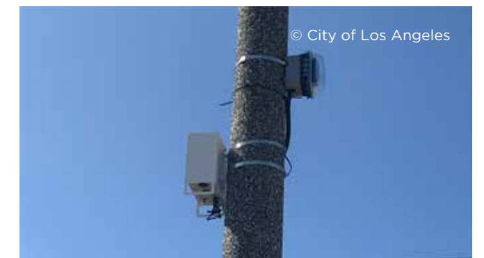
Figure 14: An Aeroqual sensor that tracks PM_{2.5} , NO_2 and O_3 installed on a city street pole in Watts.
